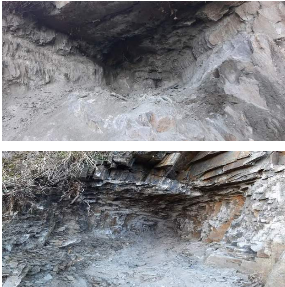
View of Excavated Material from HRT
