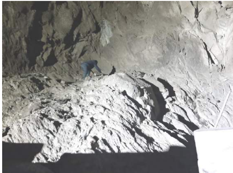
View of excavated rock material from Power House
